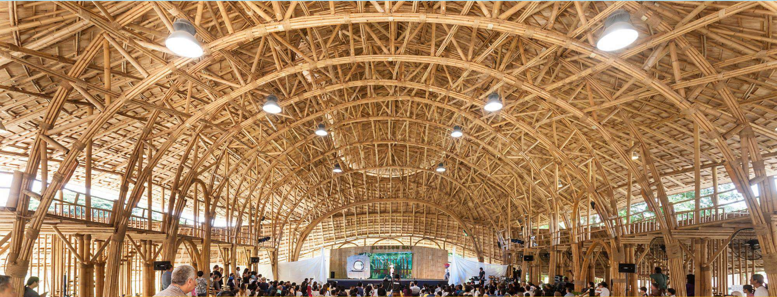
Bamboo Sports Hall of Panyaden International School (Chiang Mai, Thaïlande) - Chiangmai Life Construction
